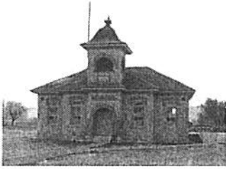
Fairfield School House, 1898
