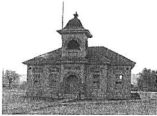
Fairfield School House, 1898
